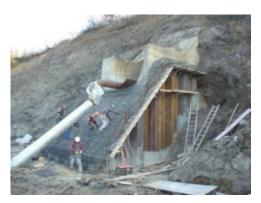
The Storm Outfall 44 Rehabilitation project consisted of rehabilitation of a 3,000 mm diameter storm outfall, including sheet piles, new concrete apron, and Class 2 rip rap erosion protection. A key feature of this project was construction of nearly a 1 km of access road within the North Saskatchewan River from Class 2 rip rap. Floating turbidity curtains were used to control sediment. The rip rap was later blended into the bank for erosion protection.
