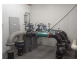
The upgrade of the City of Edmonton's Elsinore Pump Station was required to support service area expansion. This project involved a pump station preliminary design study to establish sanitary design flows and servicing options. The detailed design for pump, standby power and control upgrades is currently underway. For this project I provided project management, report preparation and process design.
